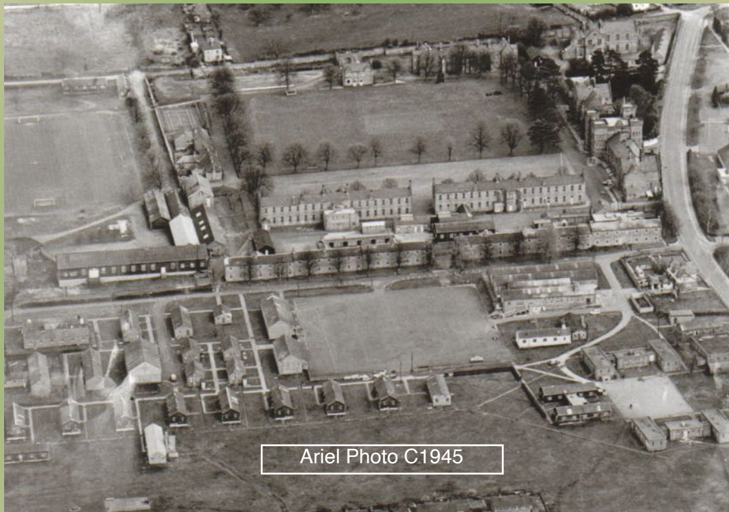
The New Building C1850
