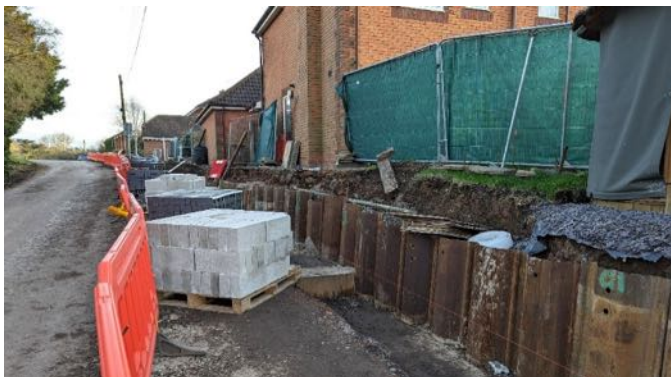
Brockhill Lane wall looking towards the Church Lane junction – 04/02/2024
