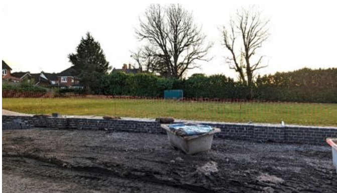
Brockhill Lane wall looking towards the Church Lane junction – 04/02/2024
